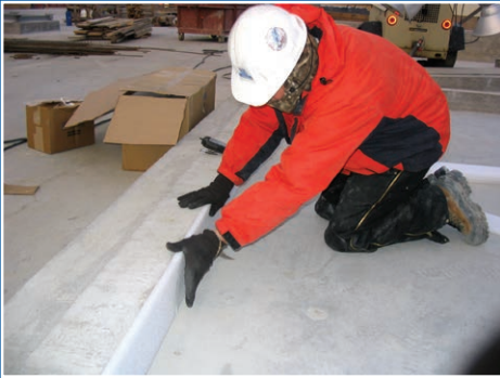
1) Place Perimeter Board (PPI)
