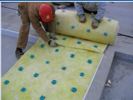
2) Roll-out RIM and cut as needed
