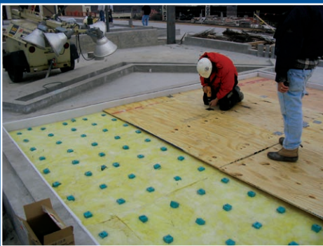
3) Secure junction plates on plywood pouring form
