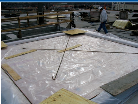
4) Cover with poly layer. Ready to install reinforcement and pour concrete.
