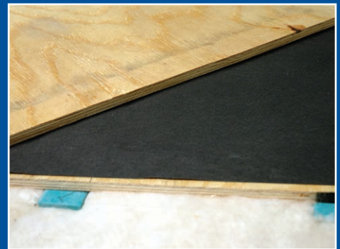
3) Build-up isolated subfloor
