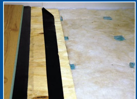
4) Apply finish floor per manufacturer instructions
