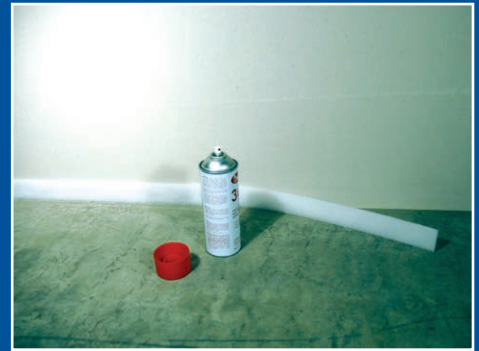
1) Place Perimeter Board (SRP)
